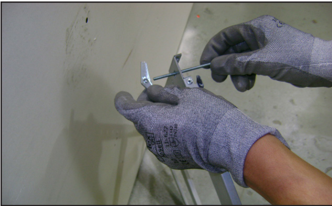
Figure 4.5 Toggle Bolt Installation through Mounting Bracket
